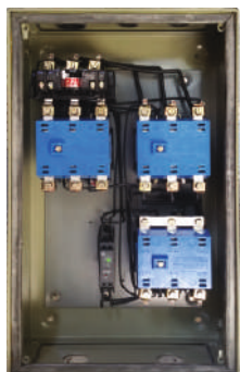
Interior View of ML FASD
