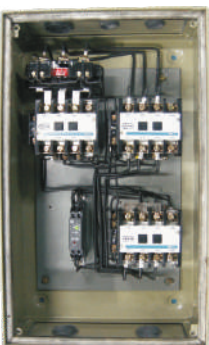
Interior View of MU FASD
